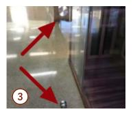
Insert the **male** door mount through the top hole in the glass door from outside the sauna, then align the **female** door mount into the male door mount.
