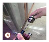
Insert the screw into the inside door mount and tighten the screw ensuring that it is snug against the glass, and not able to move or spin.
